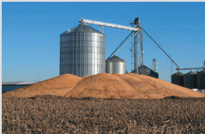
Cereal silos with bucket elevators.
